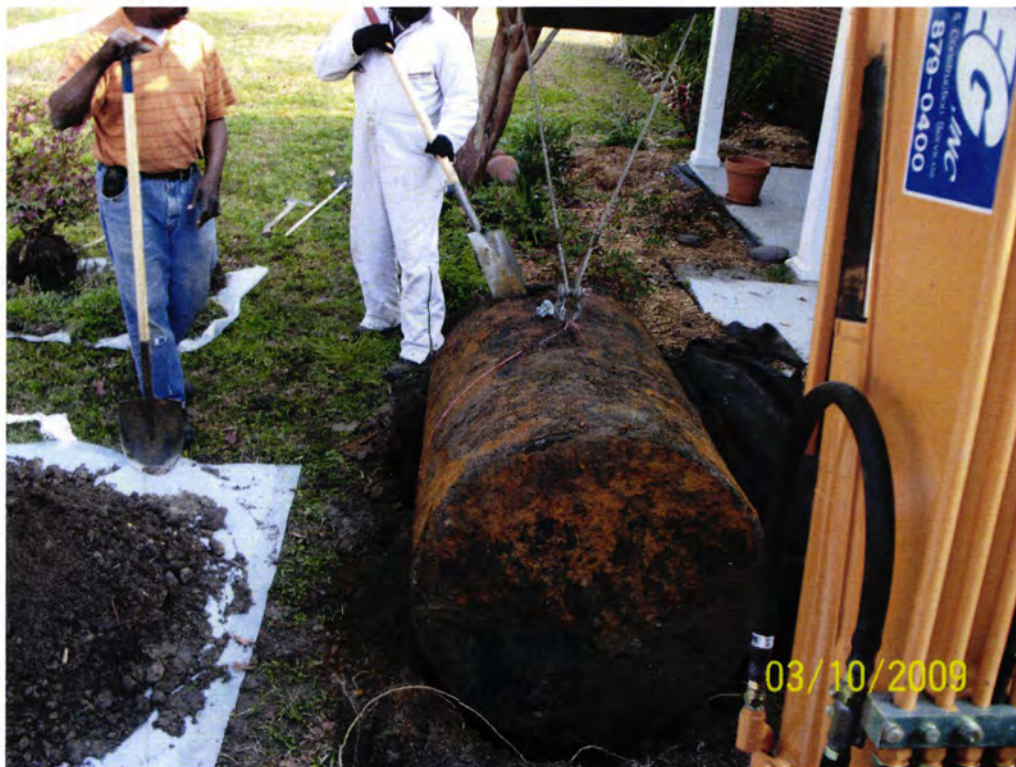
Picture 2: UST 135Birch being removed from the excavation.
